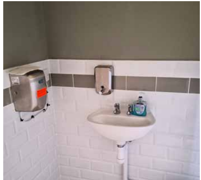
Smart looking loo: one of the newly refurbished toilets in St Michael's Church Hall. Phase Two is the outdated kitchen
